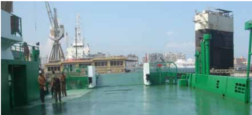
Ferry Port-Fouad; Deck painting in progress.
