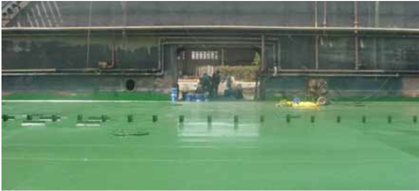
Completion of Dock floor in Transpoxy Solventfree.
