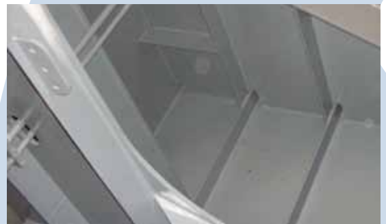
Complete renovation of Geopotes interiors with Transpoxy Masterbond.
