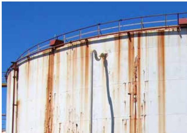
At the construction stage corrosion threats can be reduced regardless of the choice of the right protective system. Corrosion phenomena generally start in areas such as cavities or corners where water or dust are easily collected, without any drainage opportunity. A skilled designer can always change the type or the position of the sections, to avoid such drawbacks.
